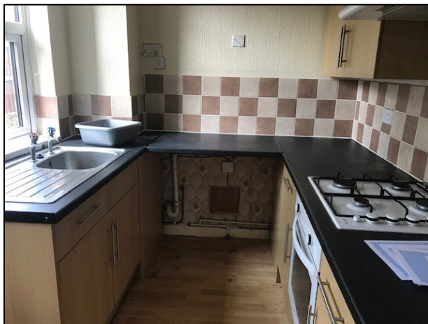
Photograph showing the existing kitchen area which will remain.
