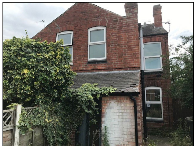
Photograph showing the rear elevation of the existing dwelling.
