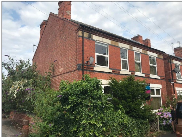
Photograph showing the front elevation of 3 Willoughby (on the left) and adjoining adjacent neighbouring property 5 Willoughby Street (on the right).
